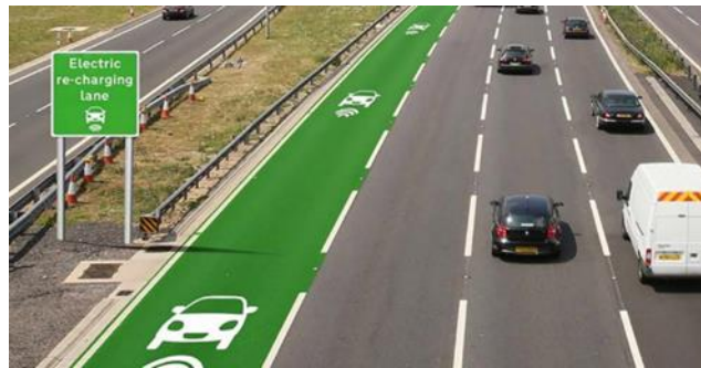
Figure 6: A dynamic charging lane on roadway
